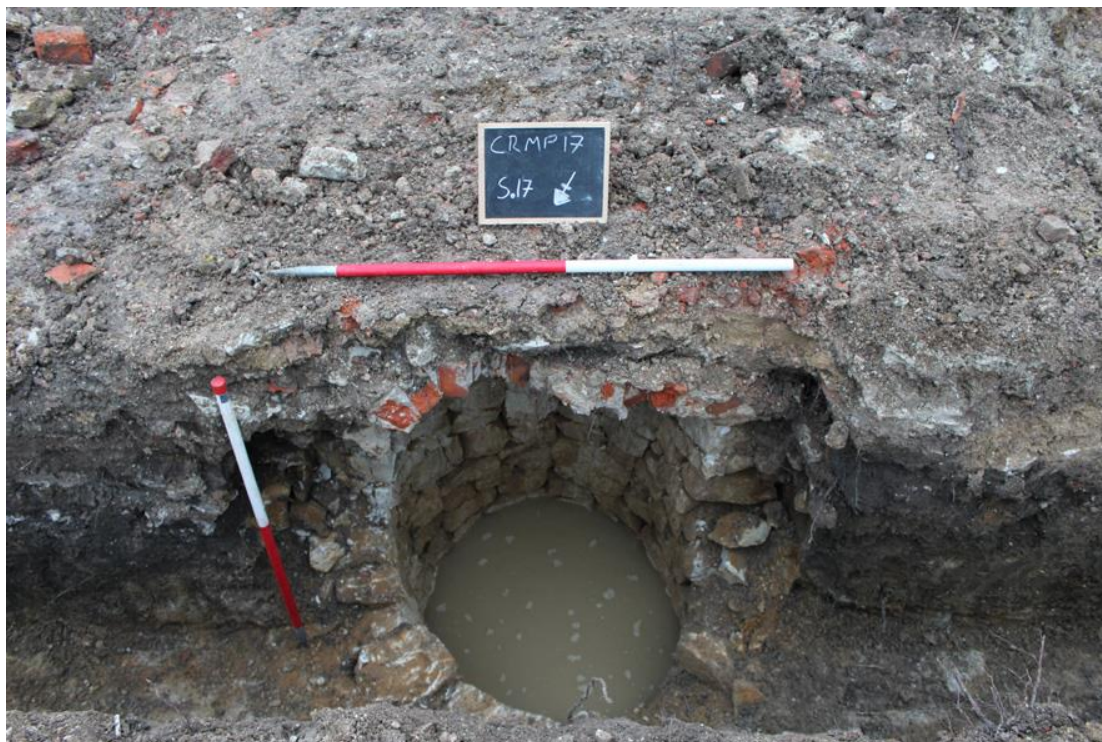
Plate 5: Chalk well 126 , seen during excavation of footings trench. Brick capping associated with Phase 4 is also evident.
