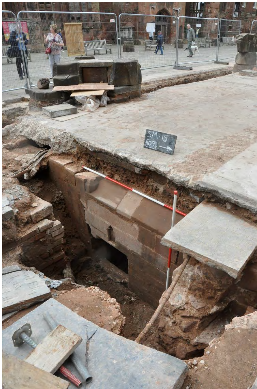
Plate 10. Wall 107. East elevation of the East Crypt. Crypt window, statue niche, buttress and bottom of the window cill for upper structure (chapel of All Saints) are visible. Pillar 103 in background, steps into crypt are just visible. View to SW.
