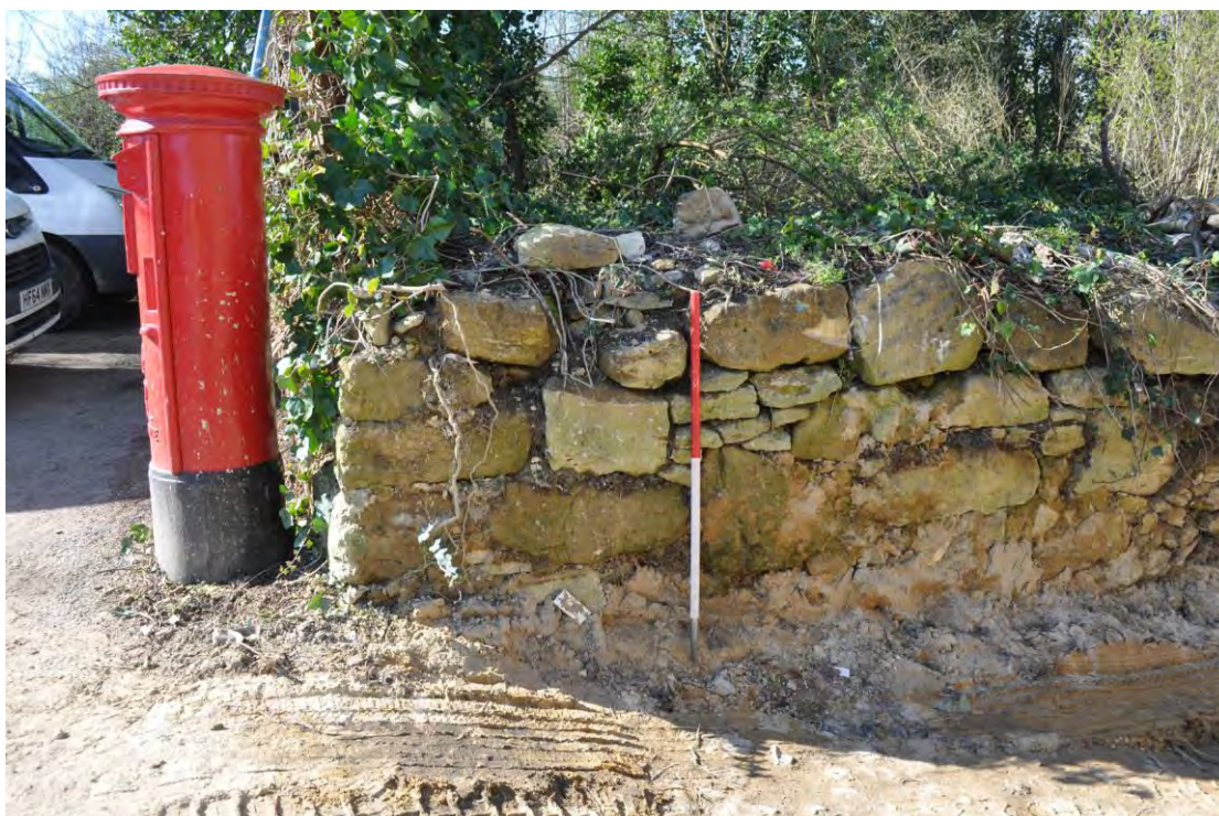
Plate 4: Quoins on south-west wall, south end
