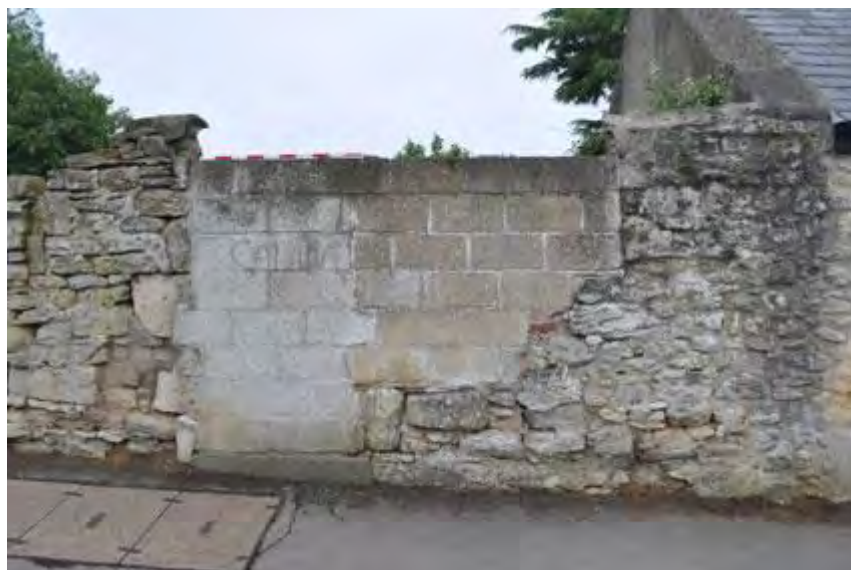
Plate 1: South-east Face of wall North Part
